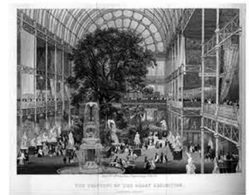
The Crystal Palace was 1,851 long and 450 feet wide. Its height of 108 feet took in some of the elm trees of Hyde Park.
